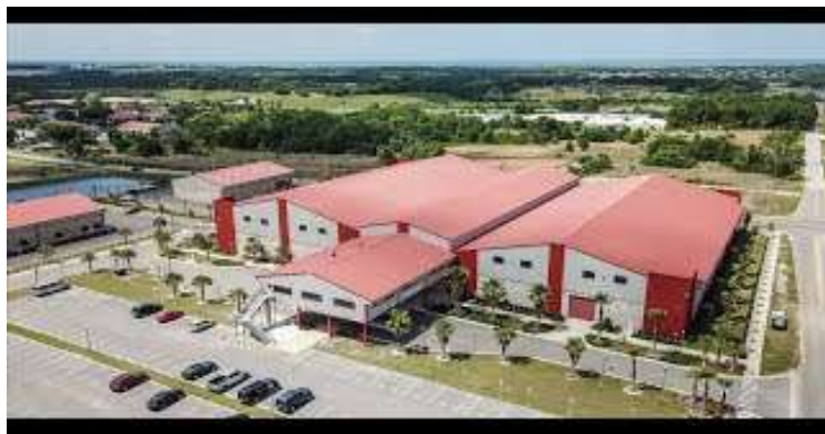
Well Activity Center- Host basketball facility.
